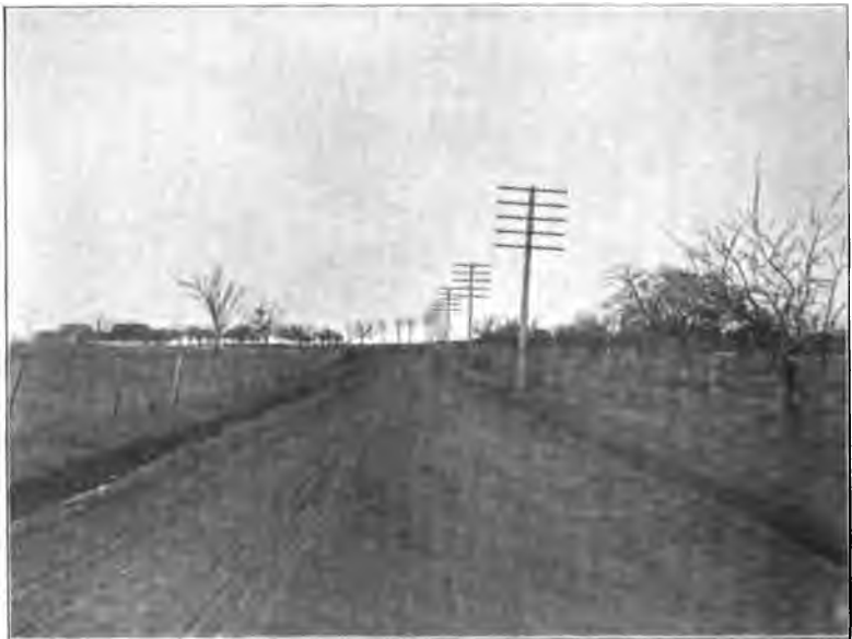
Centreville School House road, Mercer Co., after improvement.
